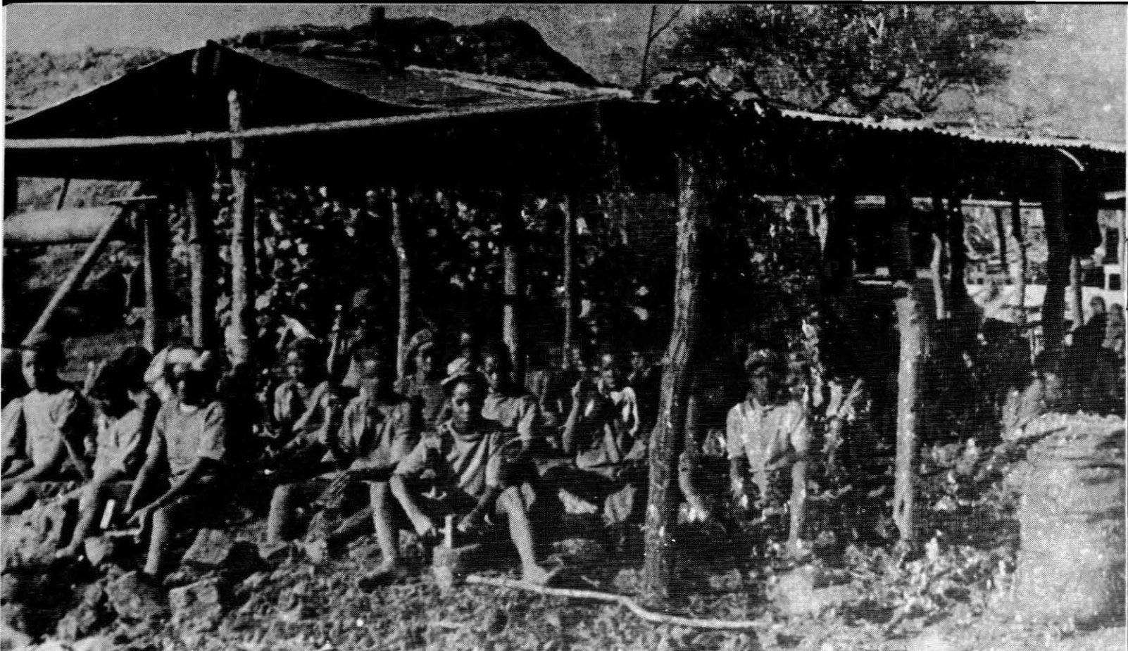
Children "cobbing" asbestos in 1917.
